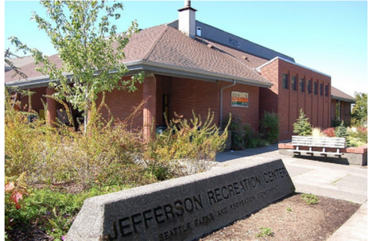
Jefferson Community Center, seismic retrofit completed in 2013
