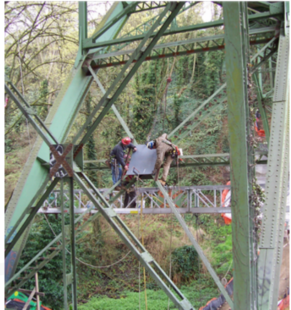
Workers complete seismic upgrades to the N Queen Anne Dr Bridge
