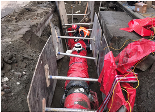
Earthquake resistant pipe installation in Pioneer Square
