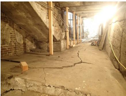
Columbia St areaway with shoring being added during the retrofit
